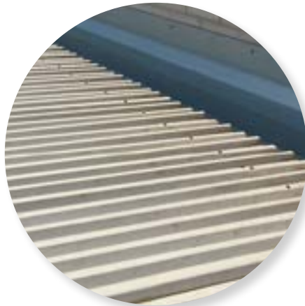
Box gutter, flashing to parapet
